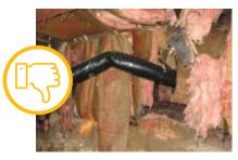
UNPREPPED CRAWL, DISCONNECTED DRYER VENT, POOR GROUND COVER Courtesy of U.S. Department of Energy
