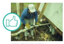
INSULATING BELLY FROM EDGE FILL METHOD Courtesy of U.S. Department of Energy
