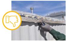
GUTTER NOT PROPERLY ATTACHED, POTENTIAL LEAKS AT ROOF EDGE
