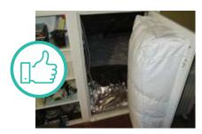
WEATHERSTRIPPED AND INSULATED HATCH Courtesy of Advanced Energyand Oregon Energy
