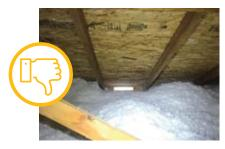
**ROOF-TO-WALL HEEL UNINSULATED**Courtesy of U.S. Department of Energy Weatherization
