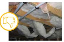
INSULATION DOES NOT FILL CAVITY AND NOT PROPERLY SUPPORTED Courtesy of ENERGY STAR, U.S. Environmental Protection Agency
