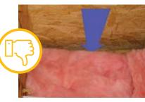
AIR GAP BETWEEN FLOOR AND INSULATION Courtesy of U.S. Department of Energy
