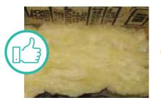
INSULATION IN FULL CONTACT WITH FLOOR Courtesy of ENERGY STAR, U.S. Environmental Protection Agency
