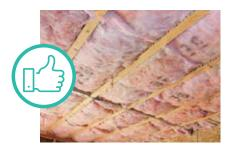
INSULATION FILLS CAVITY, PROPERLY SUPPORTED Courtesy of U.S. Department of Energy
